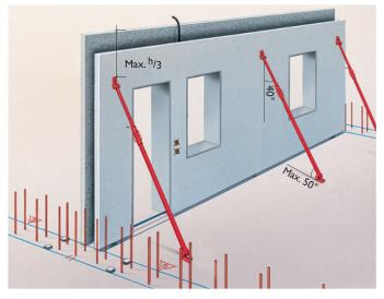
Fasten the angled supports. Then, secure them. Next, make sure they are in the correct position. Do not remove the crane hook and hook up the next wall element until these 3 steps have been completed correctly.
